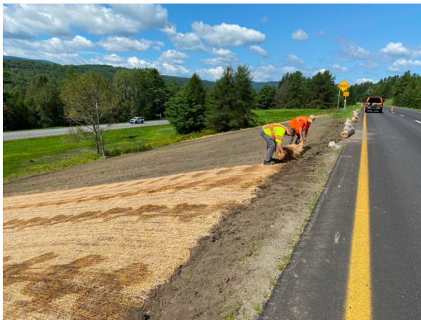
Figures 19: August 22, 2023, Digging a trench to key-in erosion control matting (left); preparing to set erosion control matting (right).
