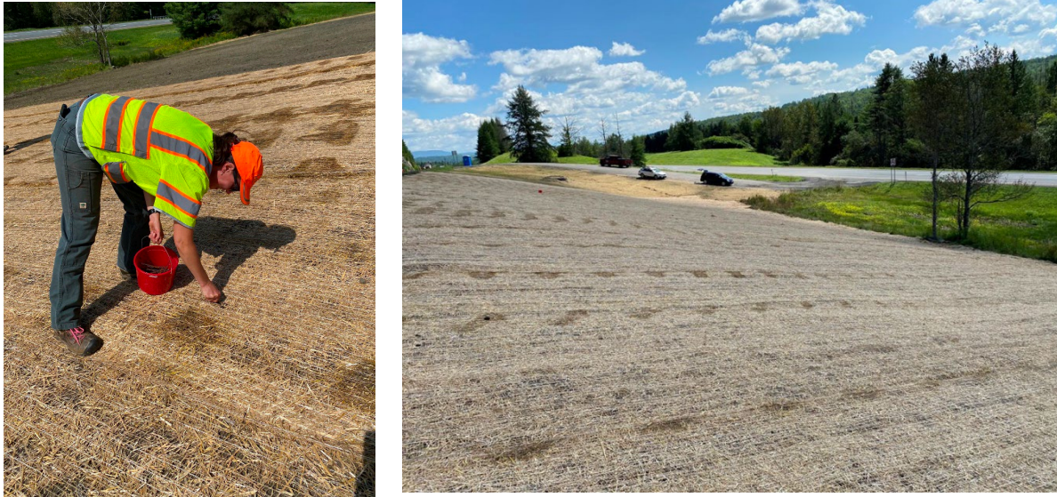
Figure 20: August 22, 2023, Installing landscape staples in matting (left); completed installation (right).
