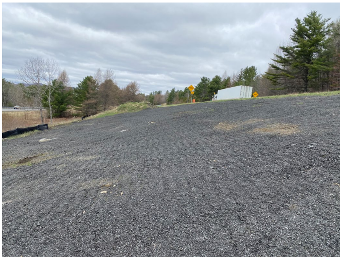
Figure 15: Asphalt millings covering site.
