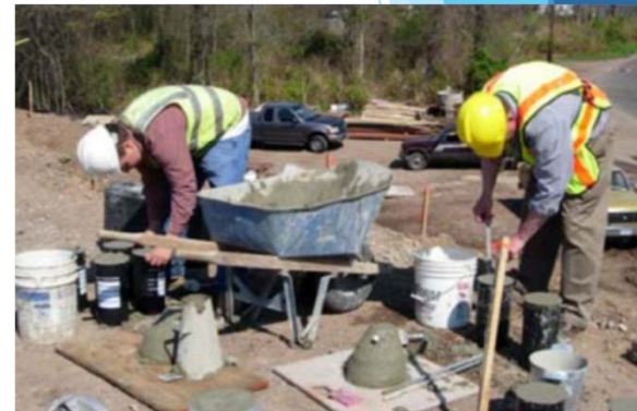
Image source: Connecticut Department of Transportation
