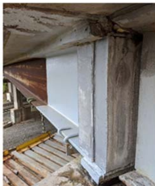
Image source: Connecticut Department of Transportation
