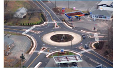
Image source: Connecticut Department of Transportation
