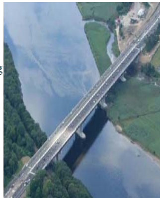
Image source: Connecticut Department of Transportation
