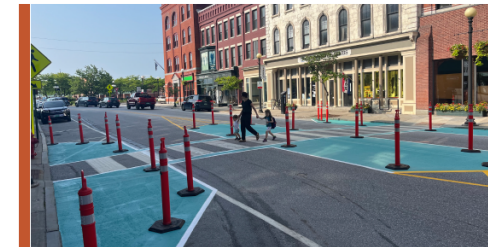
Figure 2: The median island and bollards provide refuge for pedestrians crossing a very wide street. It also narrows the traffic lanes, shortens the crossing distance, and improves conspicuity. (Credit: Rutland Regional Planning Commission)
