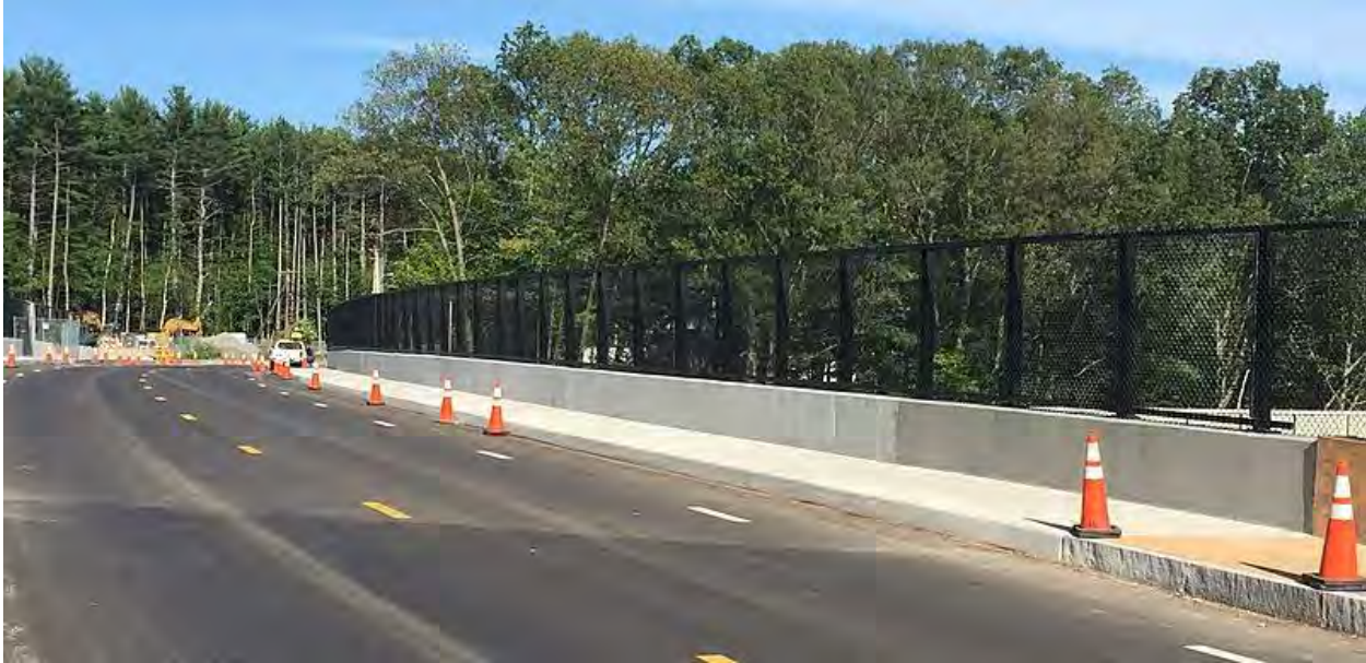
Figure 1.3 - Pine Hill Road Bridge, Newburyport, MA
