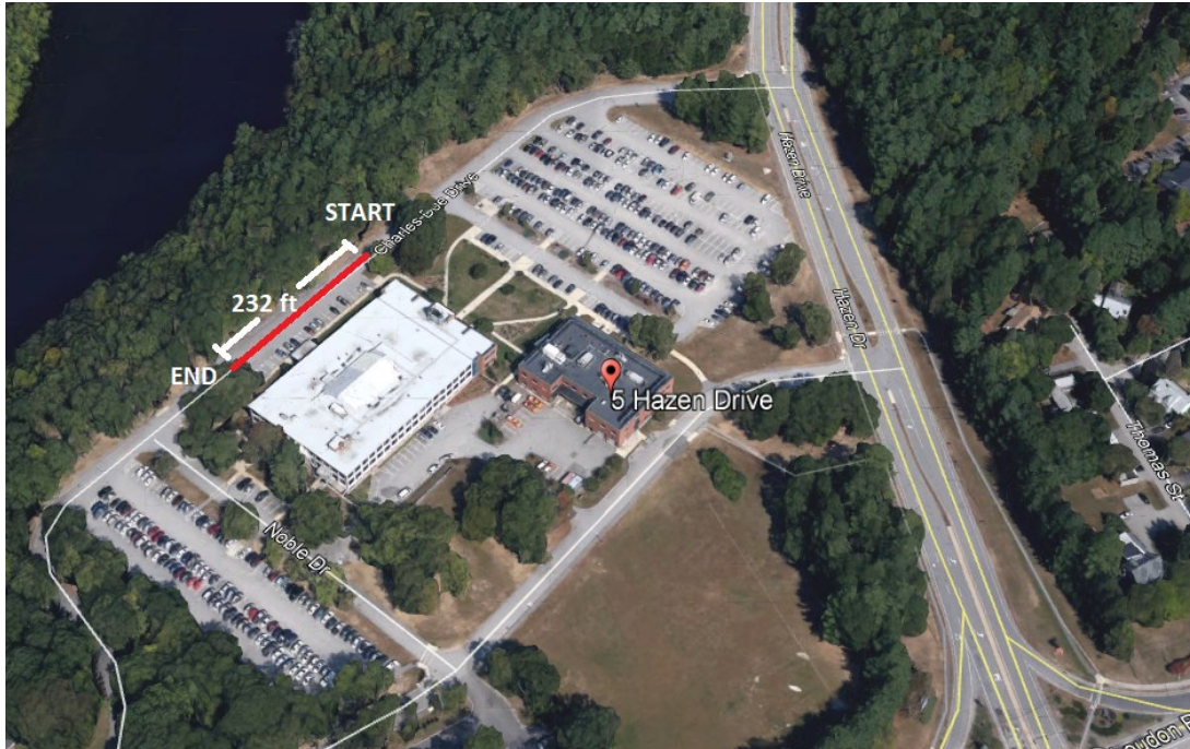
Figure 5. Fair rut & crack site at Charles Doe Drive, Concord NH, next to NHDOT office.
