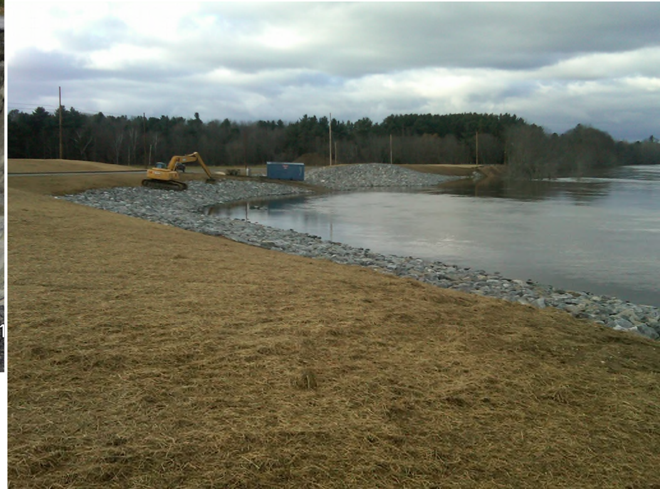
Remediated Slope December 2010
