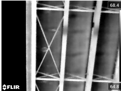
Figure 6 - Underside of Deck IR Imagery
