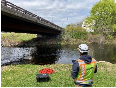
Figure 7 - UAS Bridge Inspection
