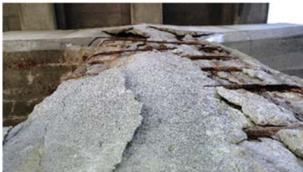
Figure 2 – Severe Delamination
