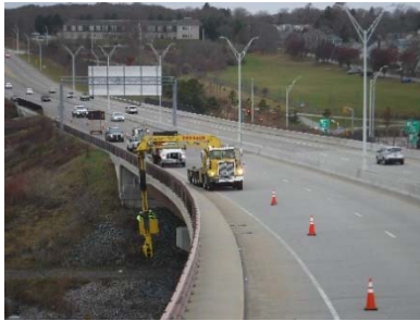
Figure 3 - Traffic Closure along Bridge
