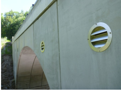
Figure 5-109: Vents on the opposite side of VT-concrete_arch
