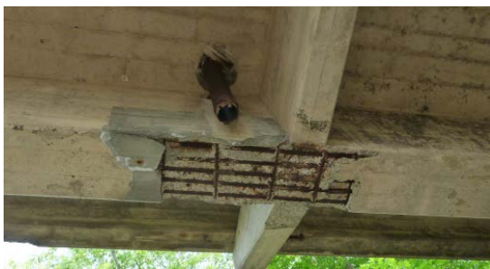
Figure 5-10: Downspouts at ME-concrete
