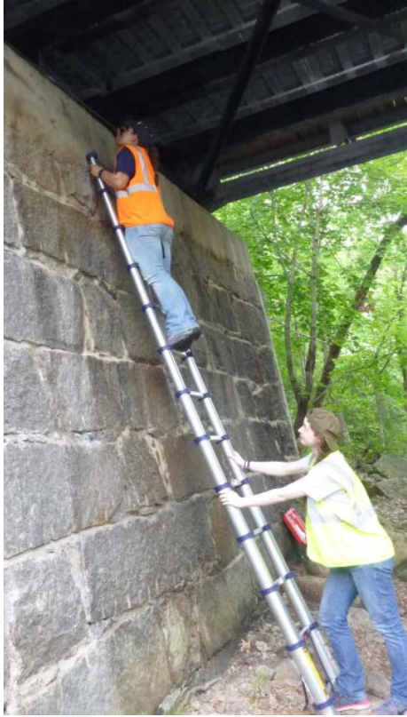
Figure 3-1: Demonstrating visual inspection of bridges utilizing a ladder and flashlight
