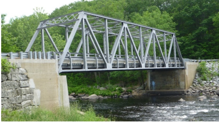
Figure 5-64: Steel truss bridge selected in NH (NH-steel_truss)
