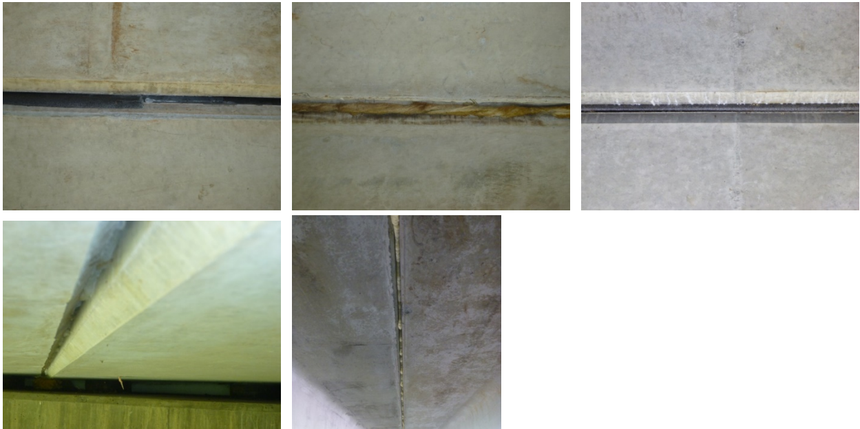
Figure 3-6: Sealed gaps between beams
