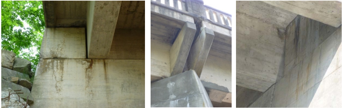
Figure 5-13: Possible roost locations at ME-concrete
