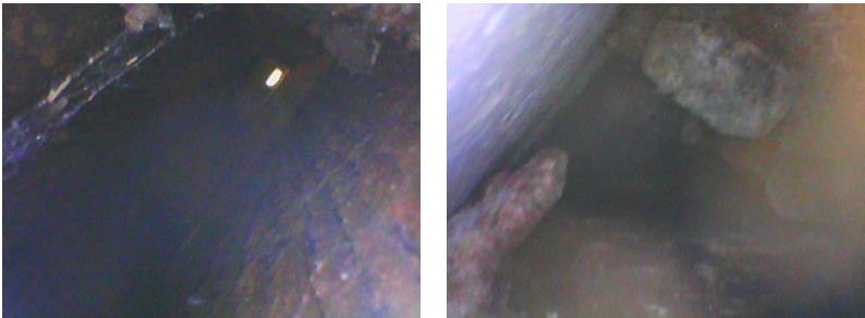
Figure 5-22: Boroscope views of spaces by the abutments at ME-steel/wood
