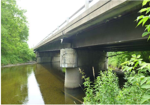
Figure 5-117: Steel construction bridge selected in VT (VT-steel)
