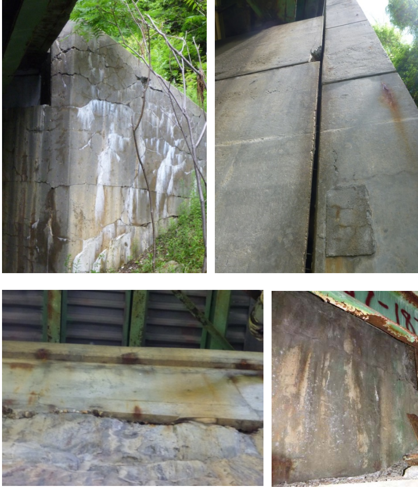
Figure 3-14: Crevices on abutments that can create suitable roosting crevices
