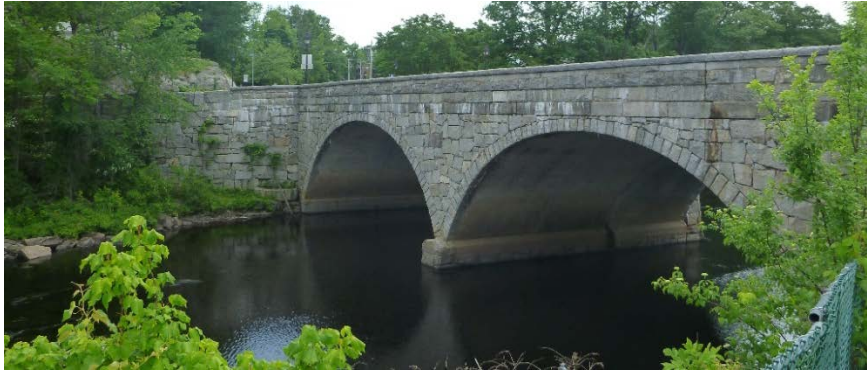
Figure 5-55: Concrete bridge selected in NH (NH-concrete_arch)
