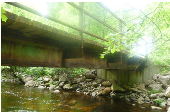
Figure 5-19: Wooden deck on steel beam construction bridge selected in ME (ME-steel/wood)
