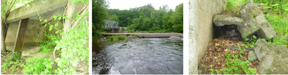
Figure 5-67: Concrete structures near NH-steel_truss
