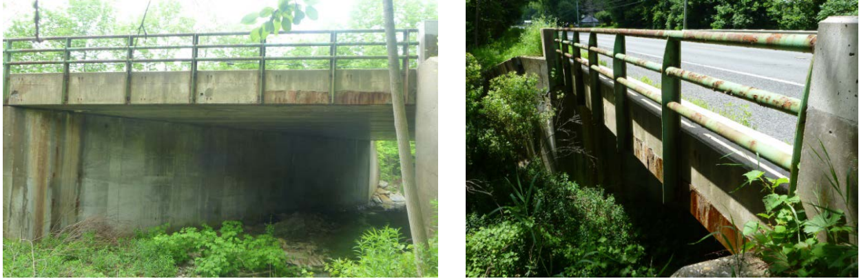
Figure 5-39: Concrete bridge selected in MA (MA-precast_concrete_2)
