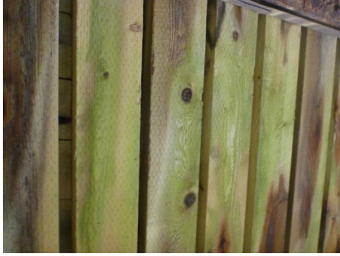
Figure 5-23: Spacing between layers of wooden decking in ME-steel/wood
