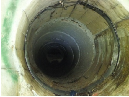
Figure 5-36: Drainage feature in MA-precast_concrete
