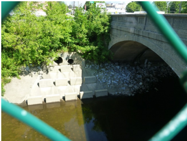
Figure 3-22: Example bridge with limited access
