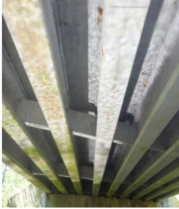
Figure 5-77: Deck construction of RI-concrete eliminating gaps and construction crevices
