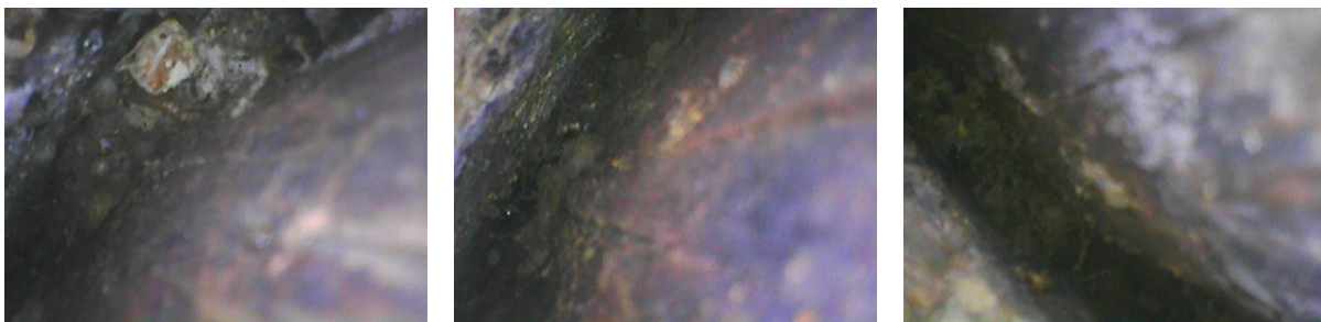
Figure 5-27: Boroscope views between deck and wooden piers at MA-concrete
