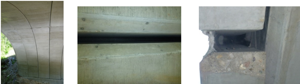
Figure 5-106: Gaps as possible roosts between segments of VT-concrete_arch
