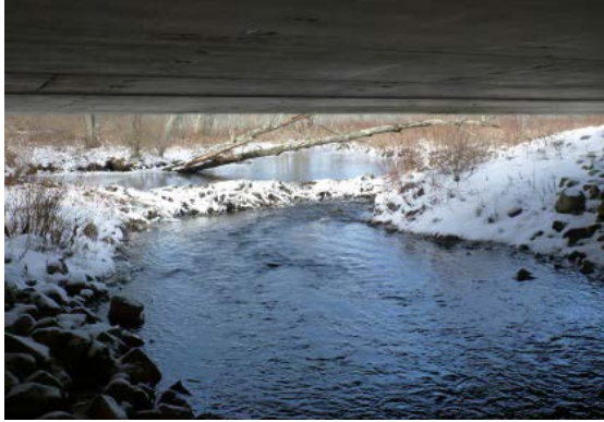
Figure 5-7: Ponded area upstream of CT-concrete
