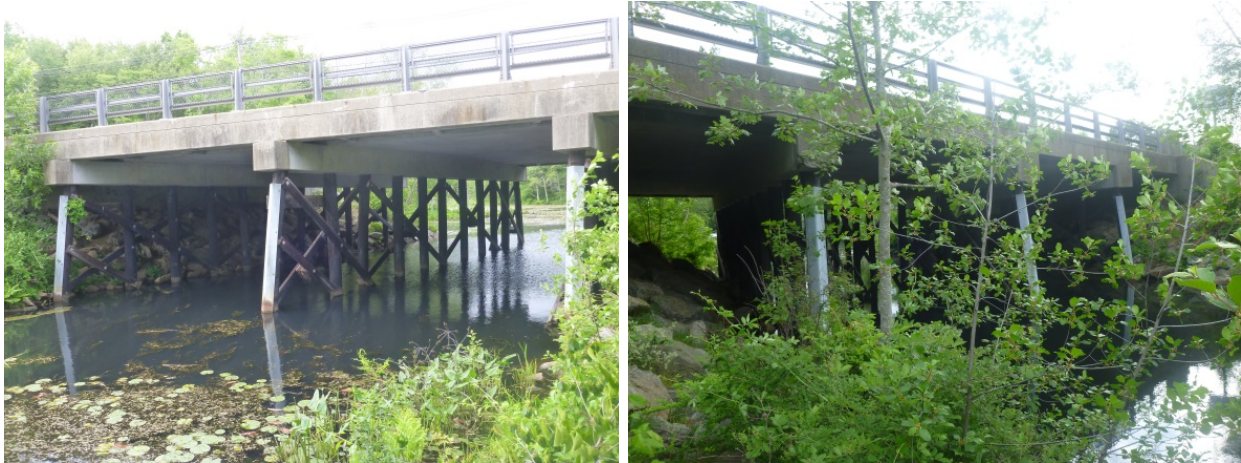
Figure 5-25: Concrete bridge selected in MA (MA-concrete)
