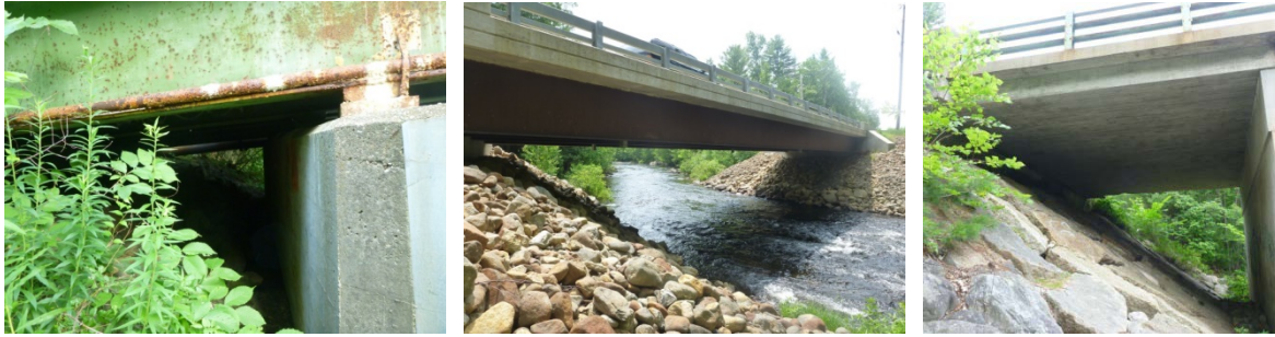
Figure 3-21: Bridge abutments with easy access by predators
