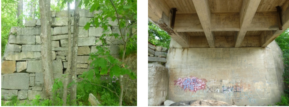
Figure 5-11: Rock partial retaining wall adjacent to the abutment at ME-concrete
