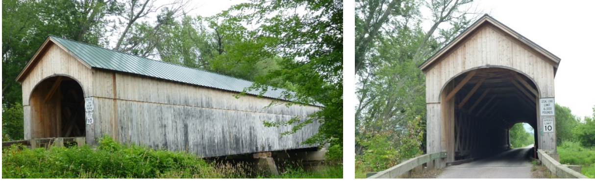
Figure 5-111: Covered wooden bridge selected in VT (VT-covered)
