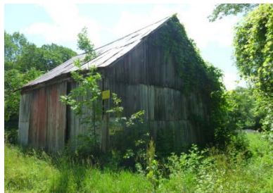
Figure 5-44: Abandoned barn near MA-precast_concrete_2
