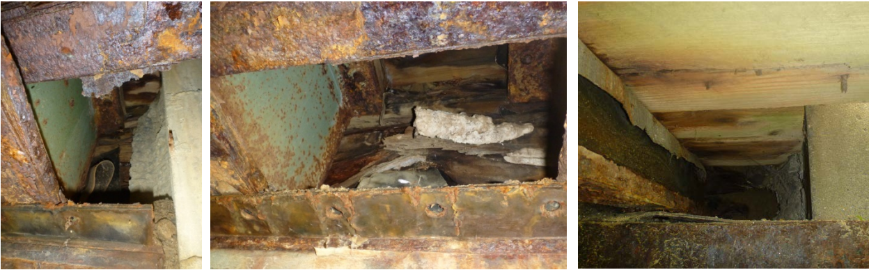
Figure 5-21: Potential roosts by the abutments in ME-steel/wood
