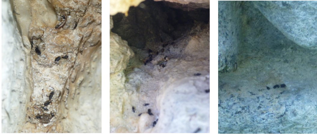
Figure 5-60: Fecal samples collected from the crevices in the stone façade at a bridge in NH-concrete_arch (assumed mouse, though unconfirmed species)
