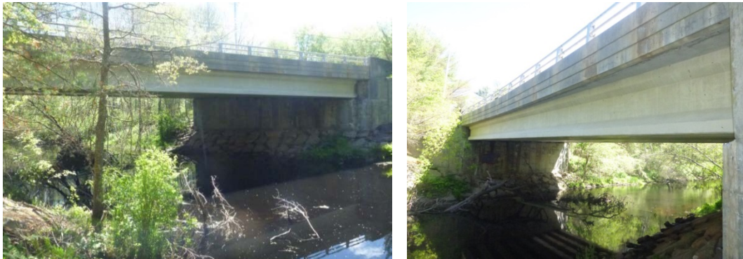
Figure 5-72: Concrete bridge selected in RI (RI-concrete)
