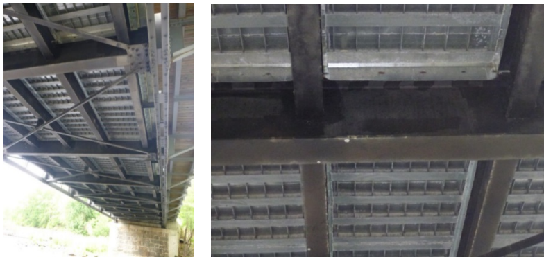
Figure 5-65: Potential open roost locations in NH-steel_truss on the uneven surfaces
