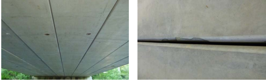
Figure 5-81: Spaces between the girders in RI-precast_concrete appropriately sized for bat roosts
