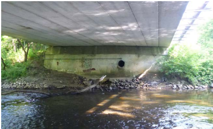
Figure 5-35: Precast concrete bridge selected in MA (MA-precast_concrete)
