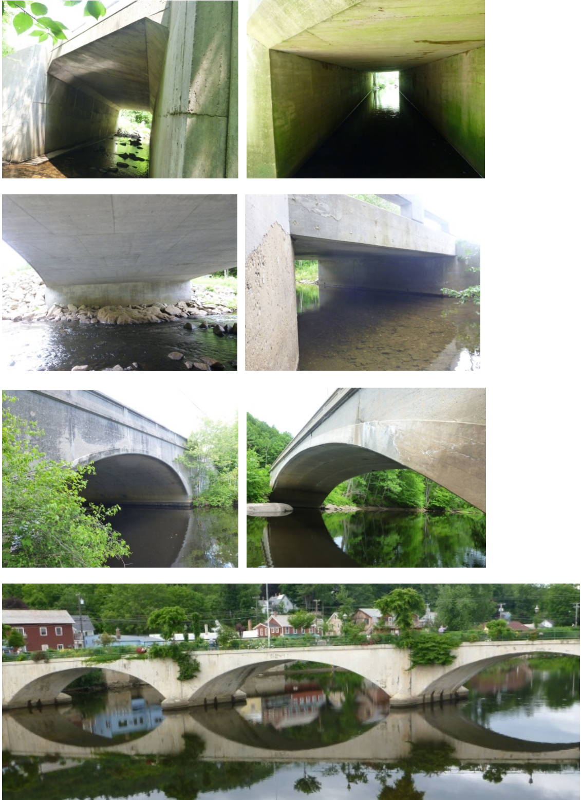
Figure 3-20: Bridges with only smooth surfaces lacking roosting locations
