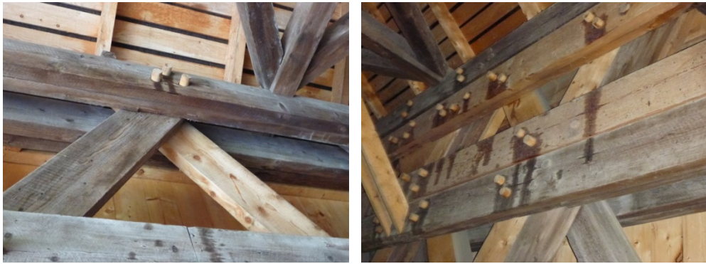
Figure 5-112: Bridge detail providing bat roost locations in VT-covered
