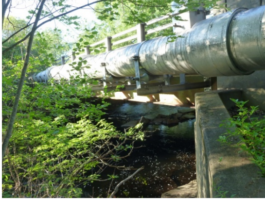
Figure 5-92: Pipes around RI-steel bridge
