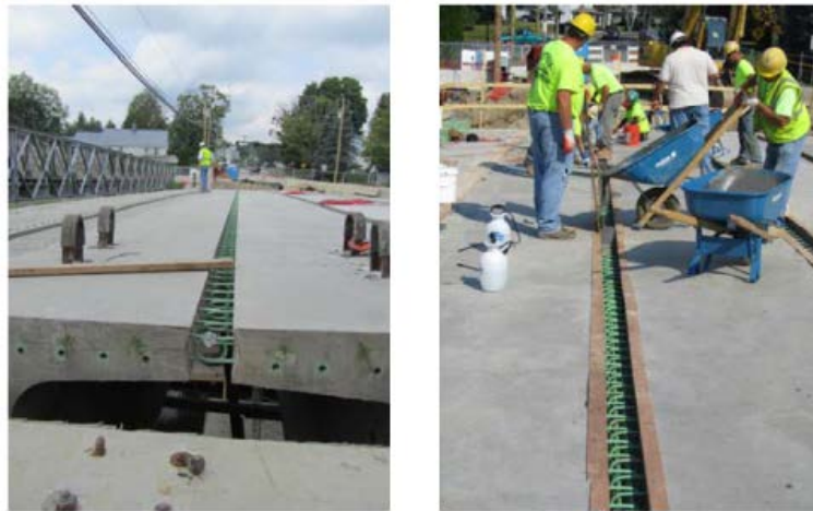
Figure 1-1: Closure pours in a Massachusetts precast bulb-tee bridge using UHPC (pictures courtesy of S. Brena)
