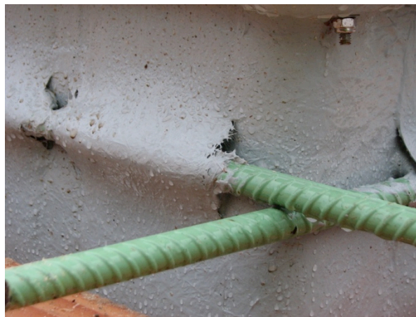
Figure 7 - Detail of drain rebar attachment (2014-12-14)
