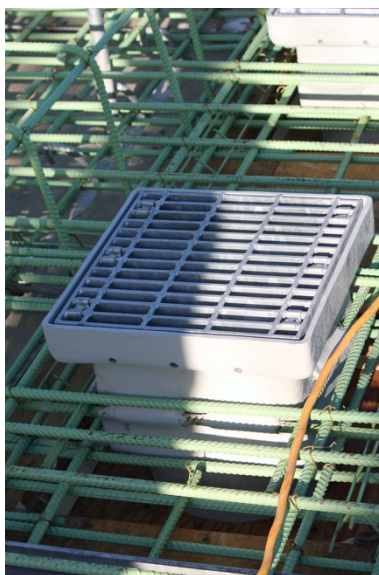
Figure 18 – Detail of grate and drain prior to concrete placement (2015-10-05)
