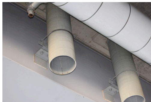
Figure 21 – Drain pipes in the westbound bridge overpass (2015-10-05)
