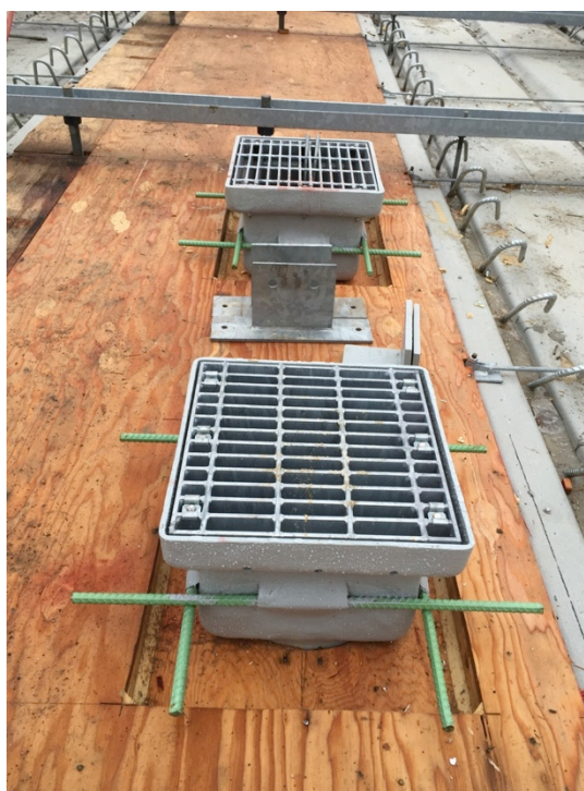
Figure 4 – Drains before concrete placement (2014-12-14)
