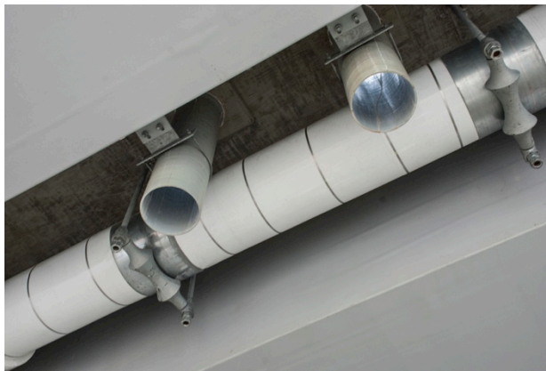
Figure 15 – Drain pipes and attachments (2015-06-03)
