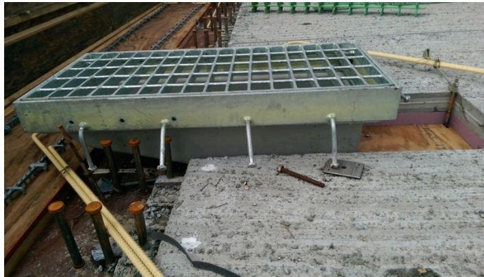
Figure 28 - Drain in place prior to rebar placement
