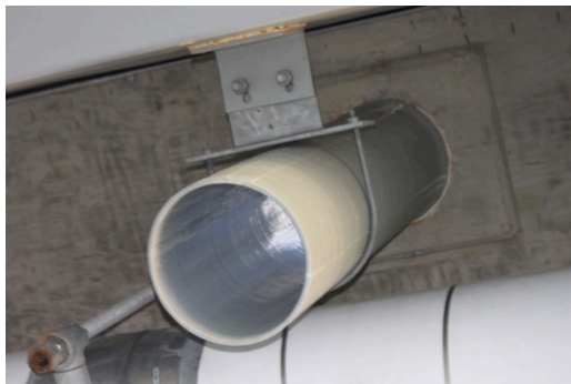
Figure 22 – Detail of drain pipe in the westbound bridge overpass (2015-10-05)
