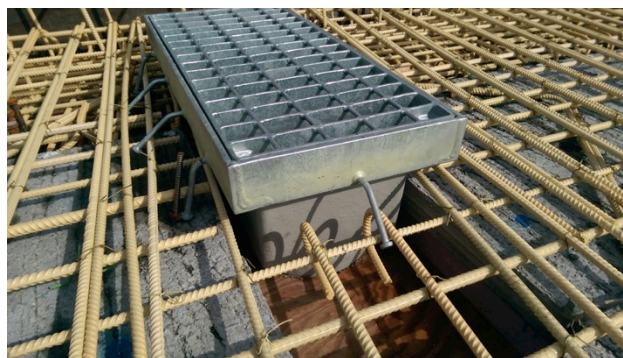
Figure 26 – Close-up of drain prior to concrete placement
