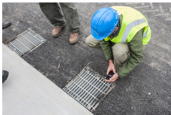
Figure 12 – Inspection of bridge drain (2015-06-03)
