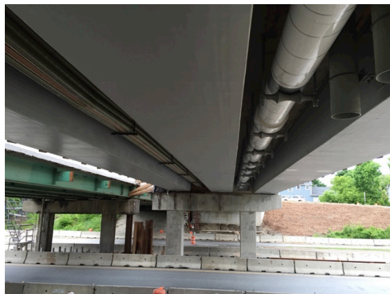
Figure 11 – Westbound bridge overpass showing drain pipes (2015-06-03)
