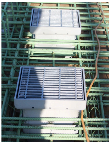
Figure 17 – Drains and slab rebar prior to concrete placement (2015-10-05)
