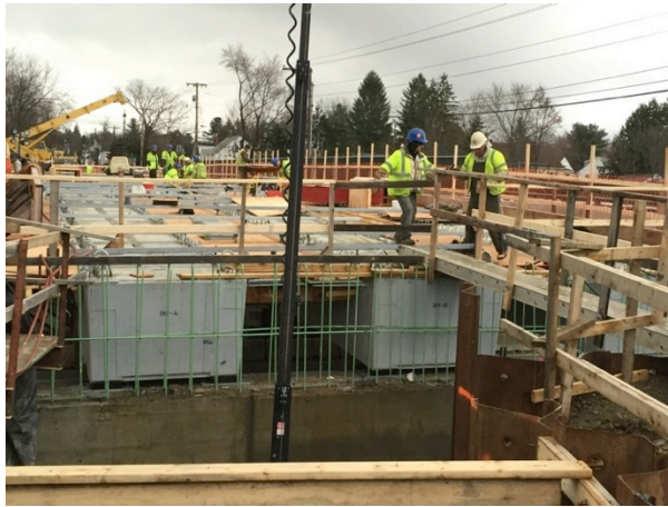
Figure 2 – HCB beams of the westbound bridge overpass (2014-12-14)
