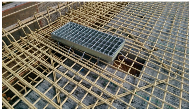
Figure 25 - Drain and slab rebar prior to concrete placement
