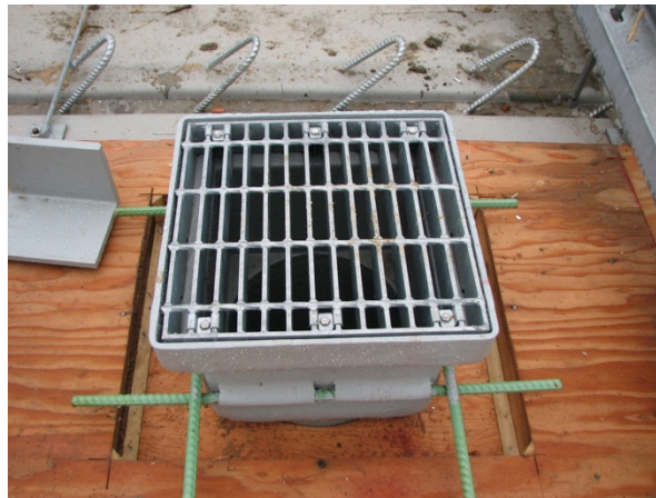
Figure 6 - Close-up of drain prior to concrete placement (2014-12-14)
