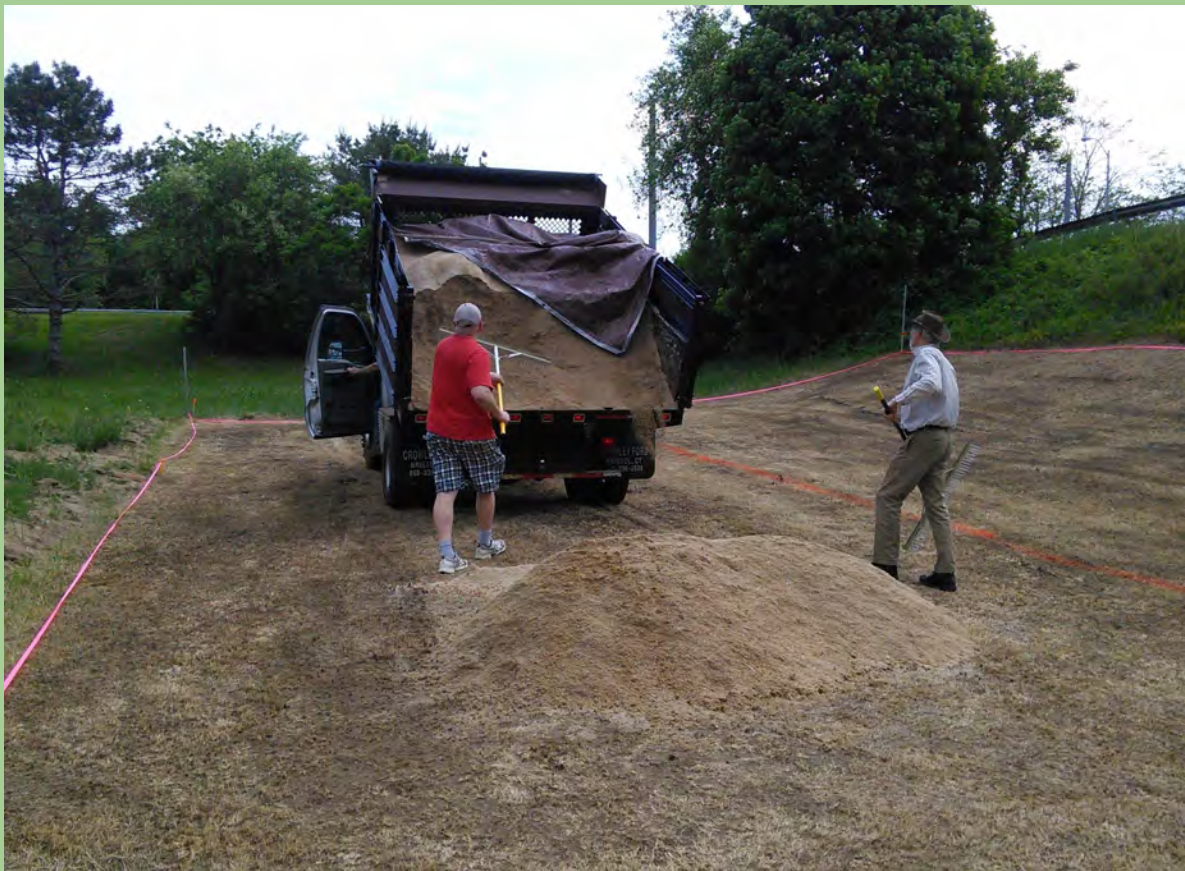
Figure 3.9 Sawdust brought to site along US Route 6 using a dump truck.
