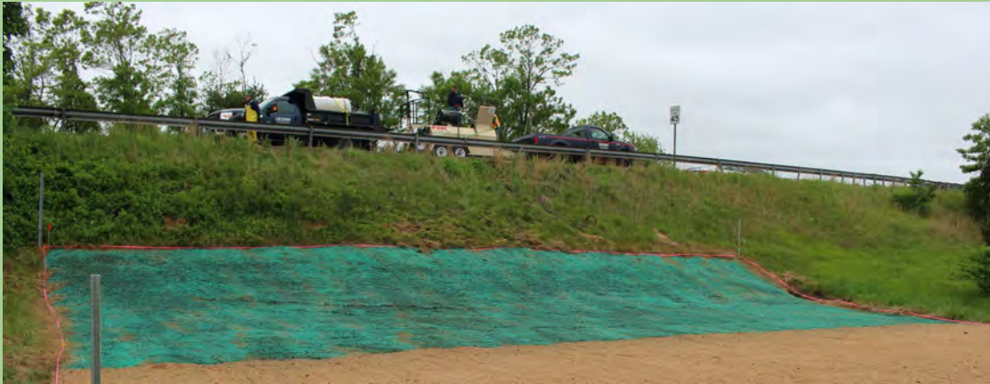
Figure 3.6 Hydroseeded slope along US Route 6.
